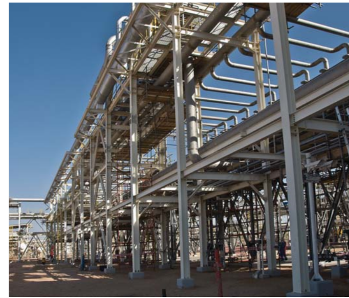
A view from under the Pipe Rack
