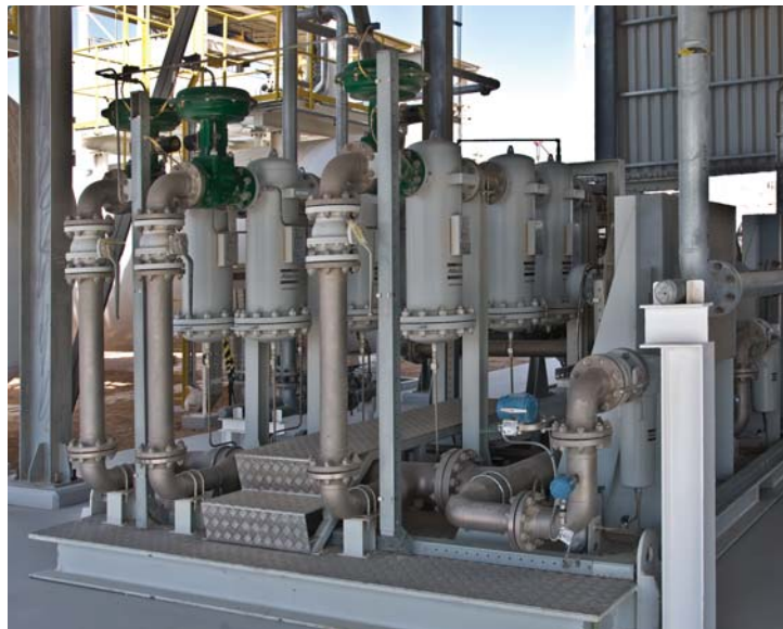
Instrument Air Shelter
