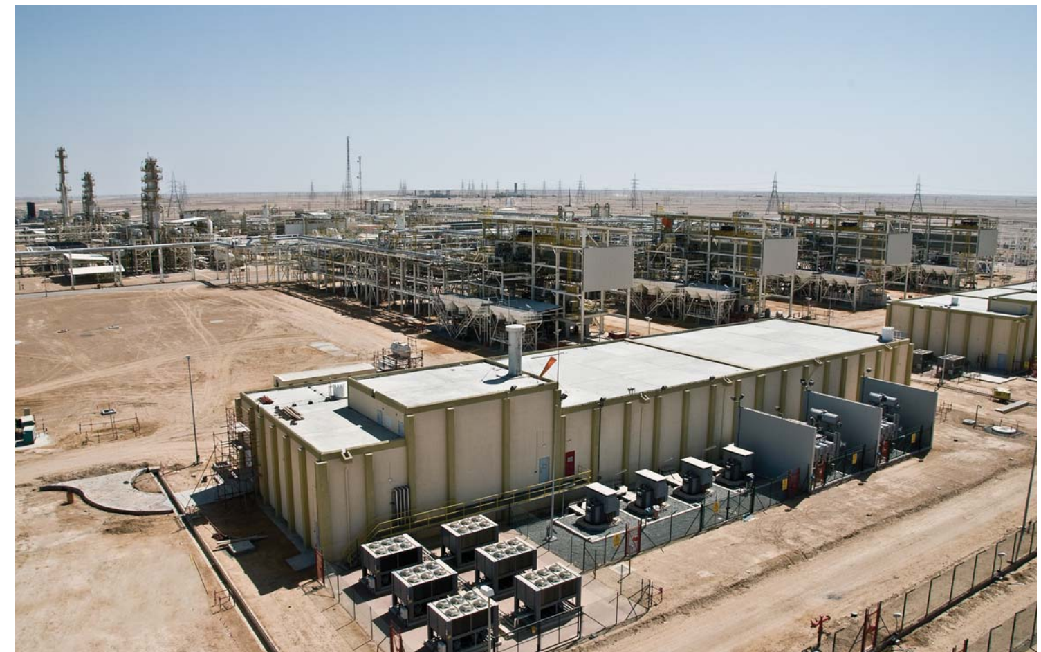
Aerial view of Compression Plant
