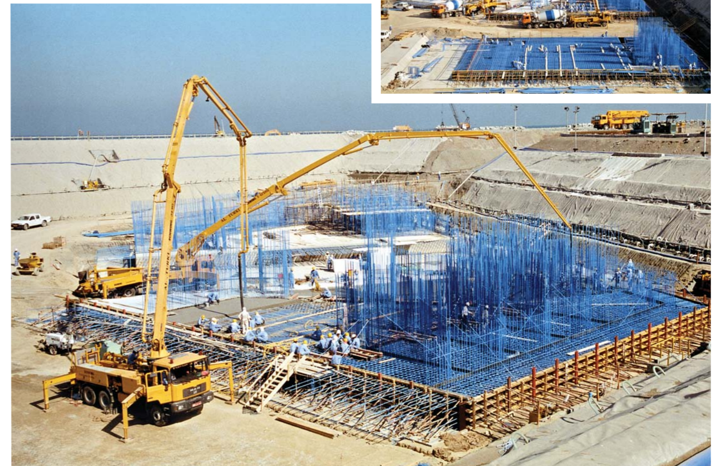
Bottom & Inset: Raft Concreting in progress
