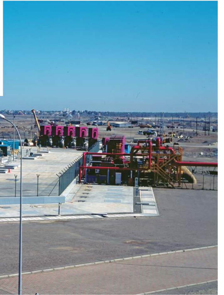
Bottom: Finished Pumping Station
