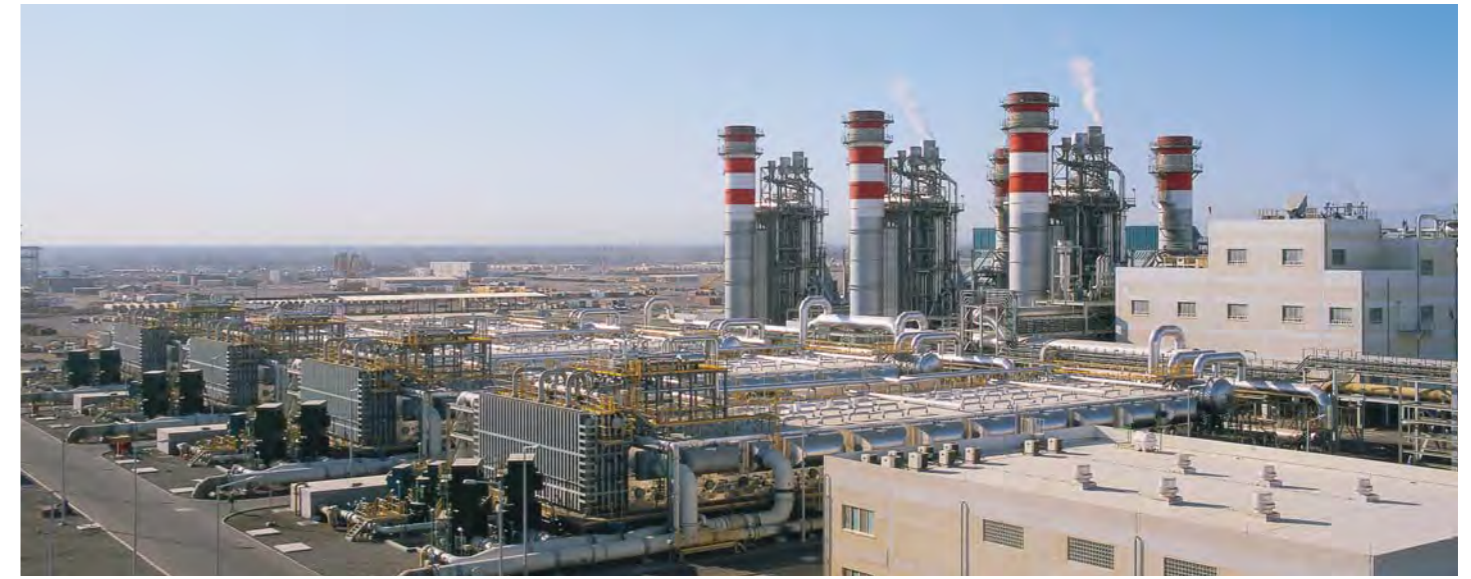
IWPP Sohar – Desal Unit in the foreground
