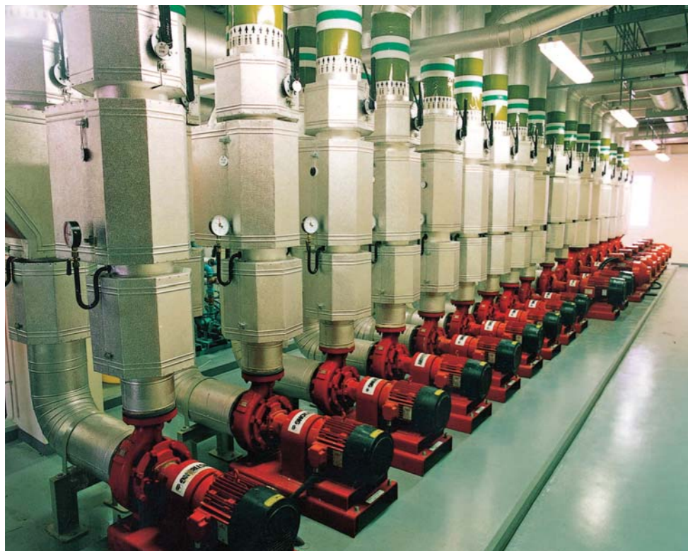
Pumps Installation in Mechanical Plant Room
