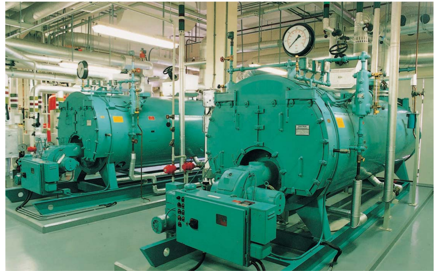
Boilers and Steam Piping Installation
