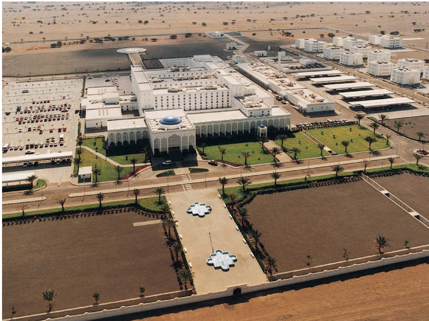
Mechanical, Electrical Services for 380 Bed Hospital and Residential Complex – Sohar
