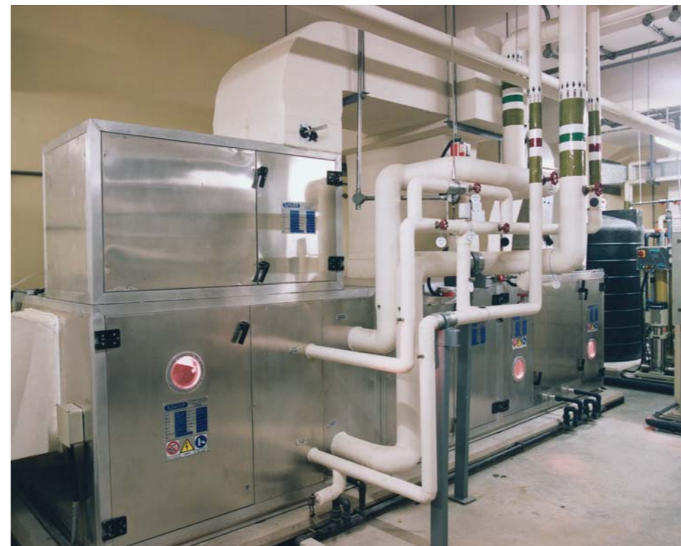
Air Handling Unit Installation
