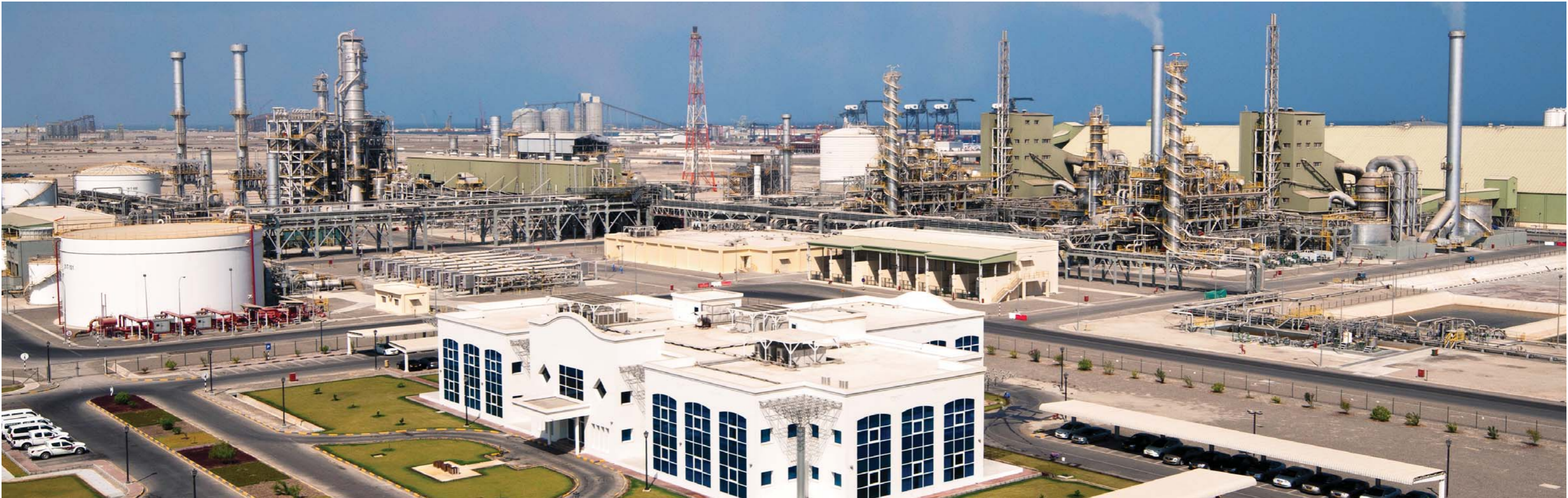
Panoramic view of the Plant
