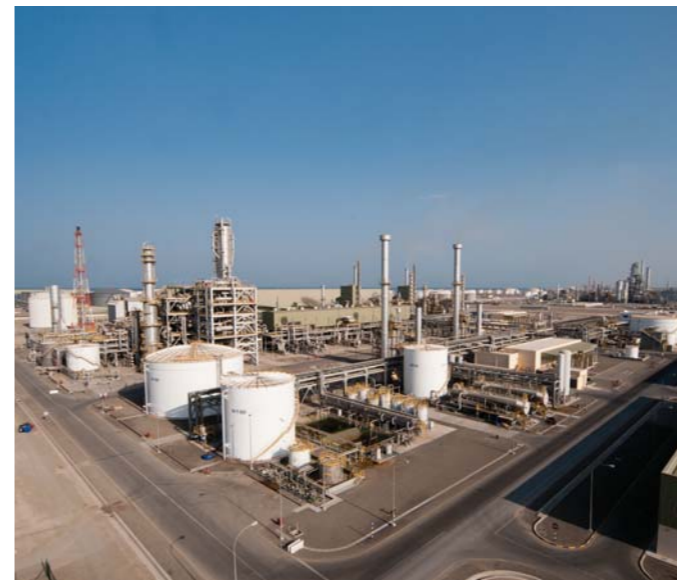
Utility area overlooking the Ammonia plant
