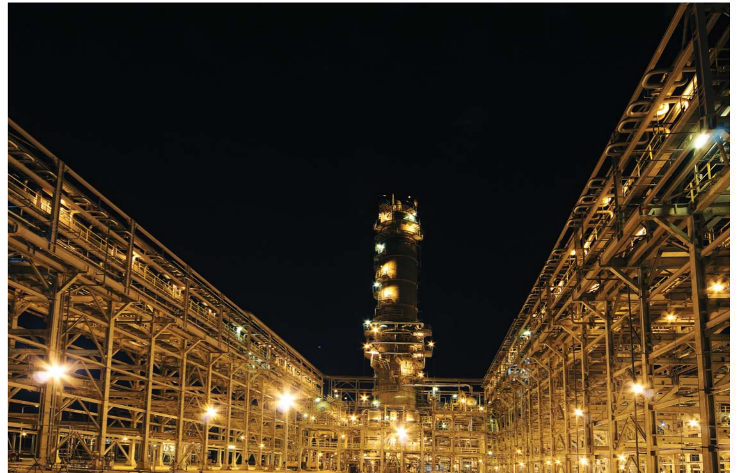
Heavy Ends Column & Piperack
