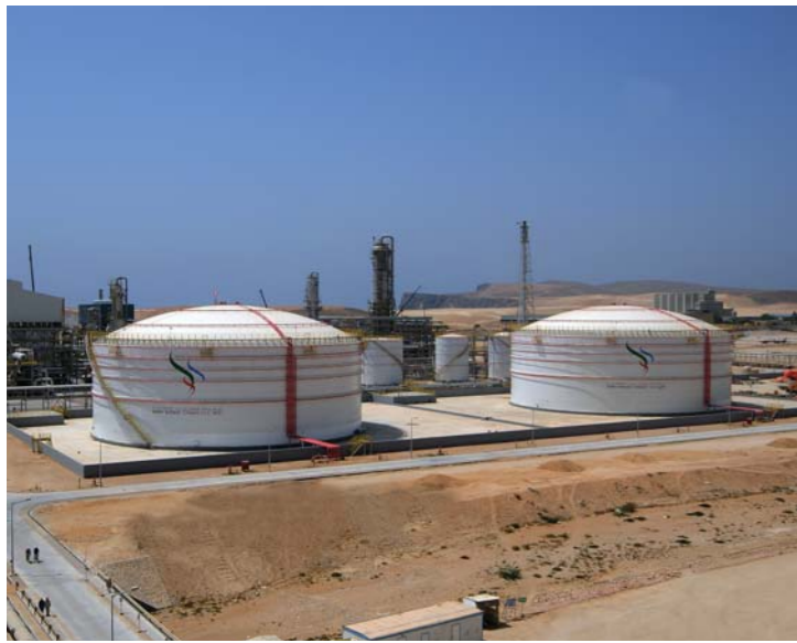
Methanol Storage Tank
