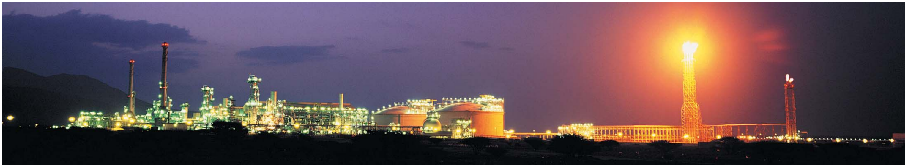
Panoramic night view of the Oman LNG Plant
