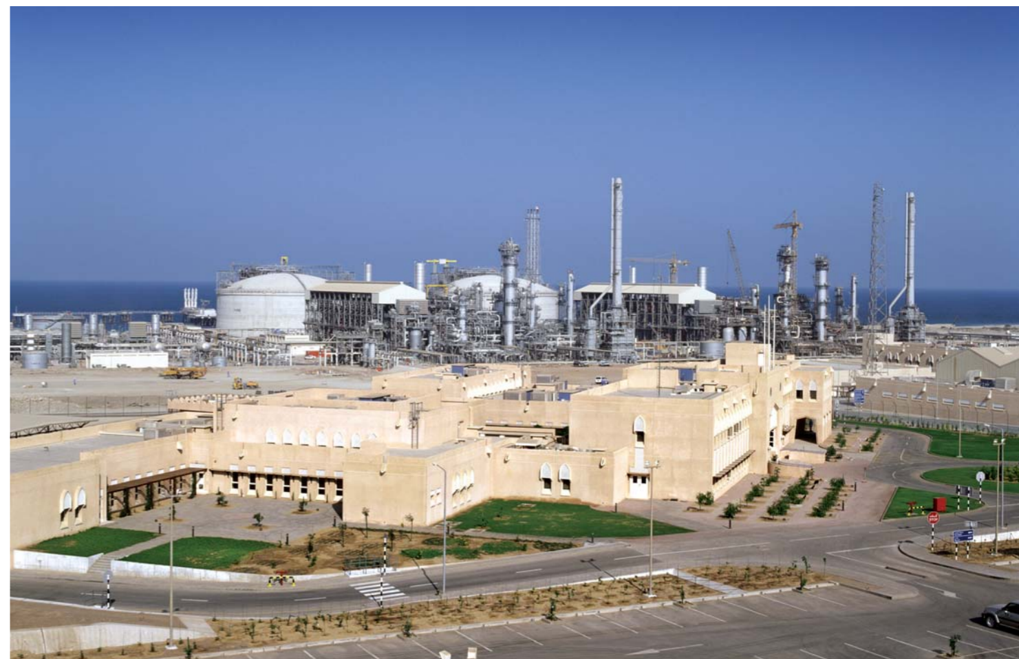
Overall view of Oman LNG Plant with the Non-Industrial Buildings in the foreground
