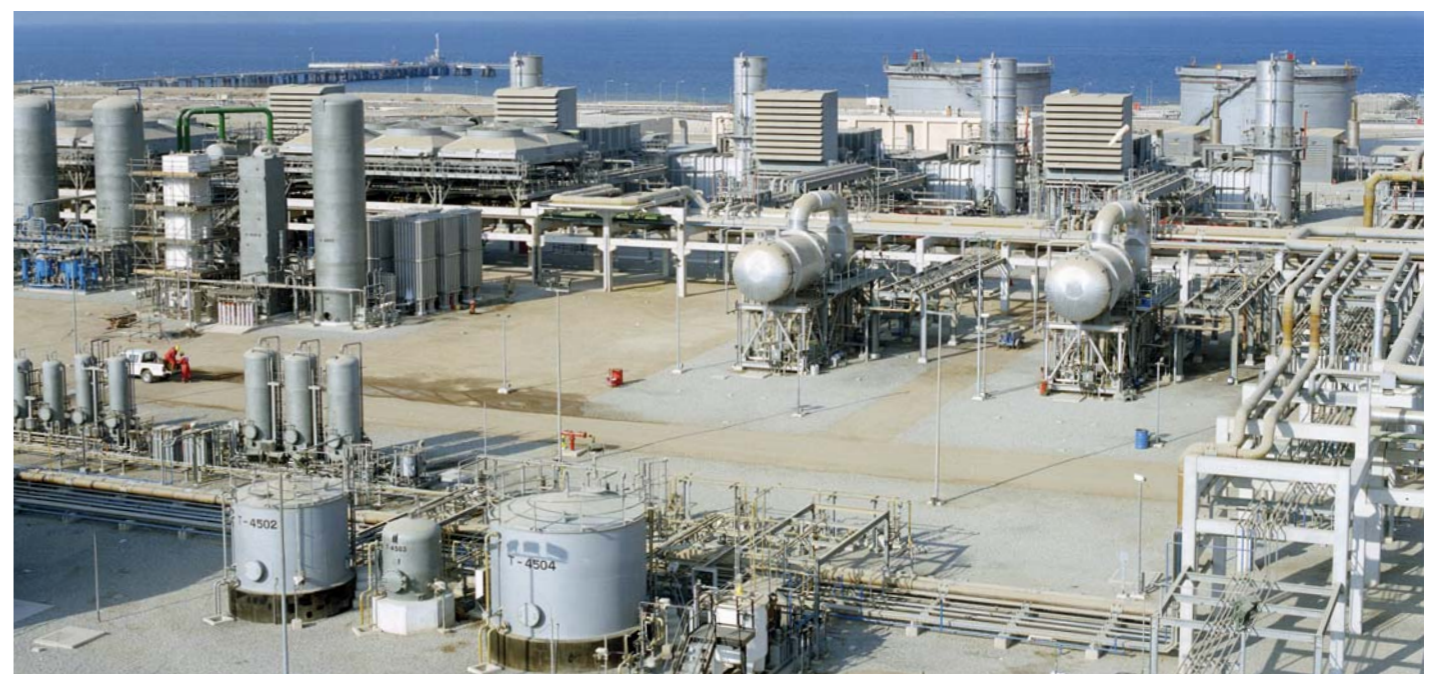
View of the Oman LNG Plant Utility Area
