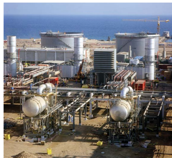
1200 M 3 / day Desalination Plant
