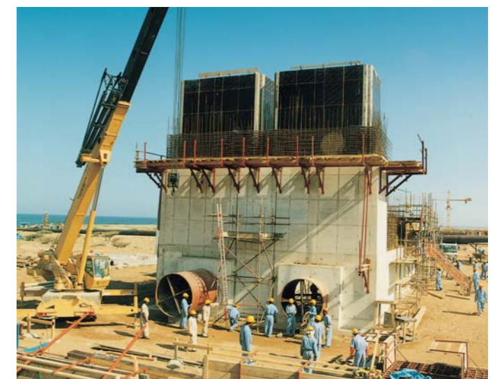
Sea Water outlet weir structure
