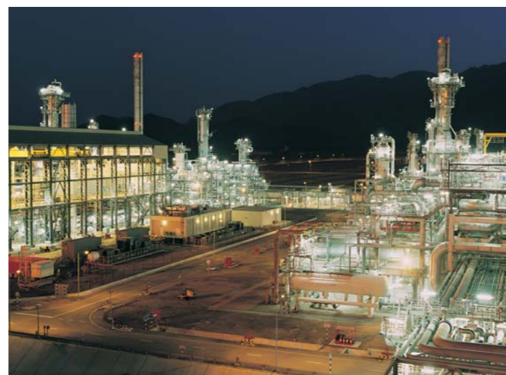
Electrical & Instrumentation works for the Process Plant.
