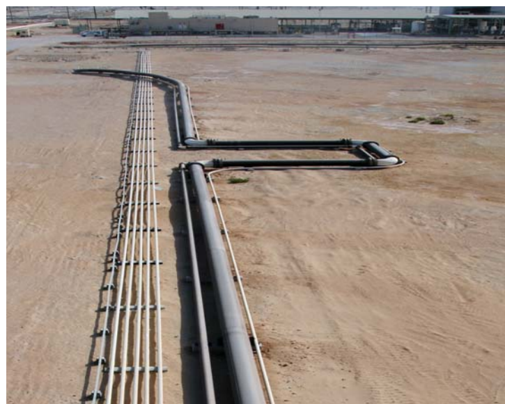
Off-plot Flowlines and Pipelines
