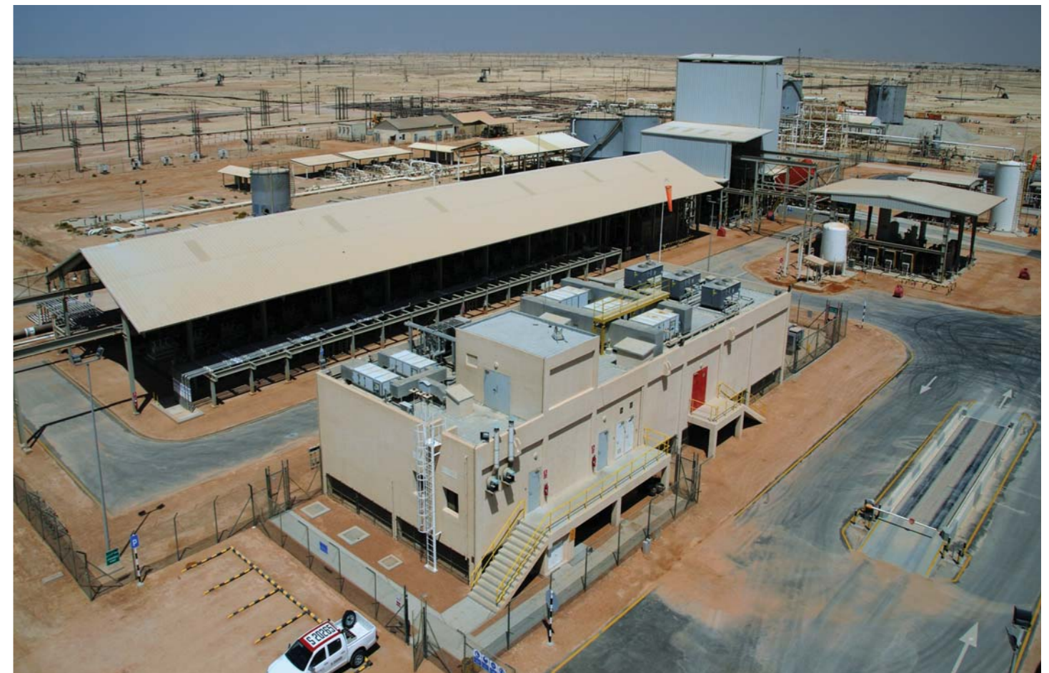
Polymer Plant and Control Room Overview
