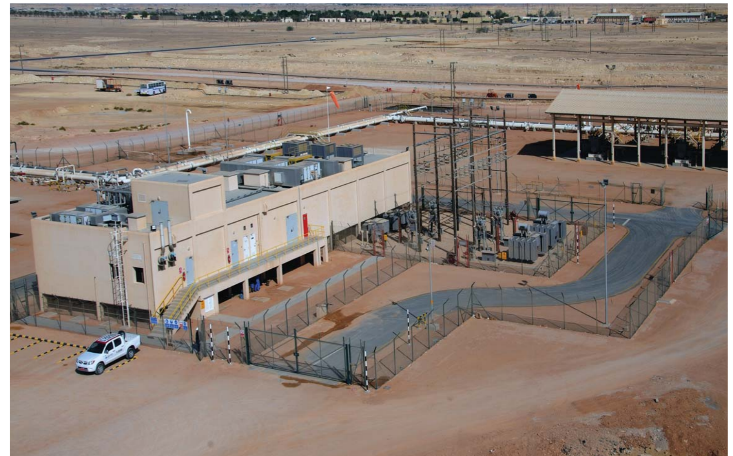
Water Treatment Plant Control Room and Power Transformers
