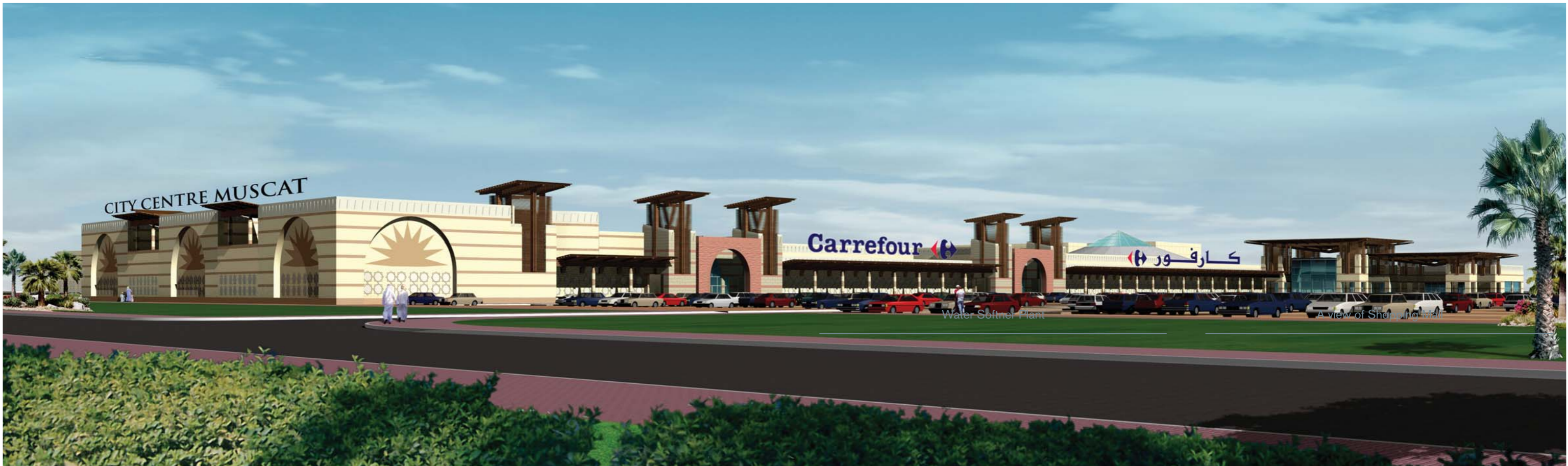
Mechanical and Electrical Services for City Centre – Muscat
