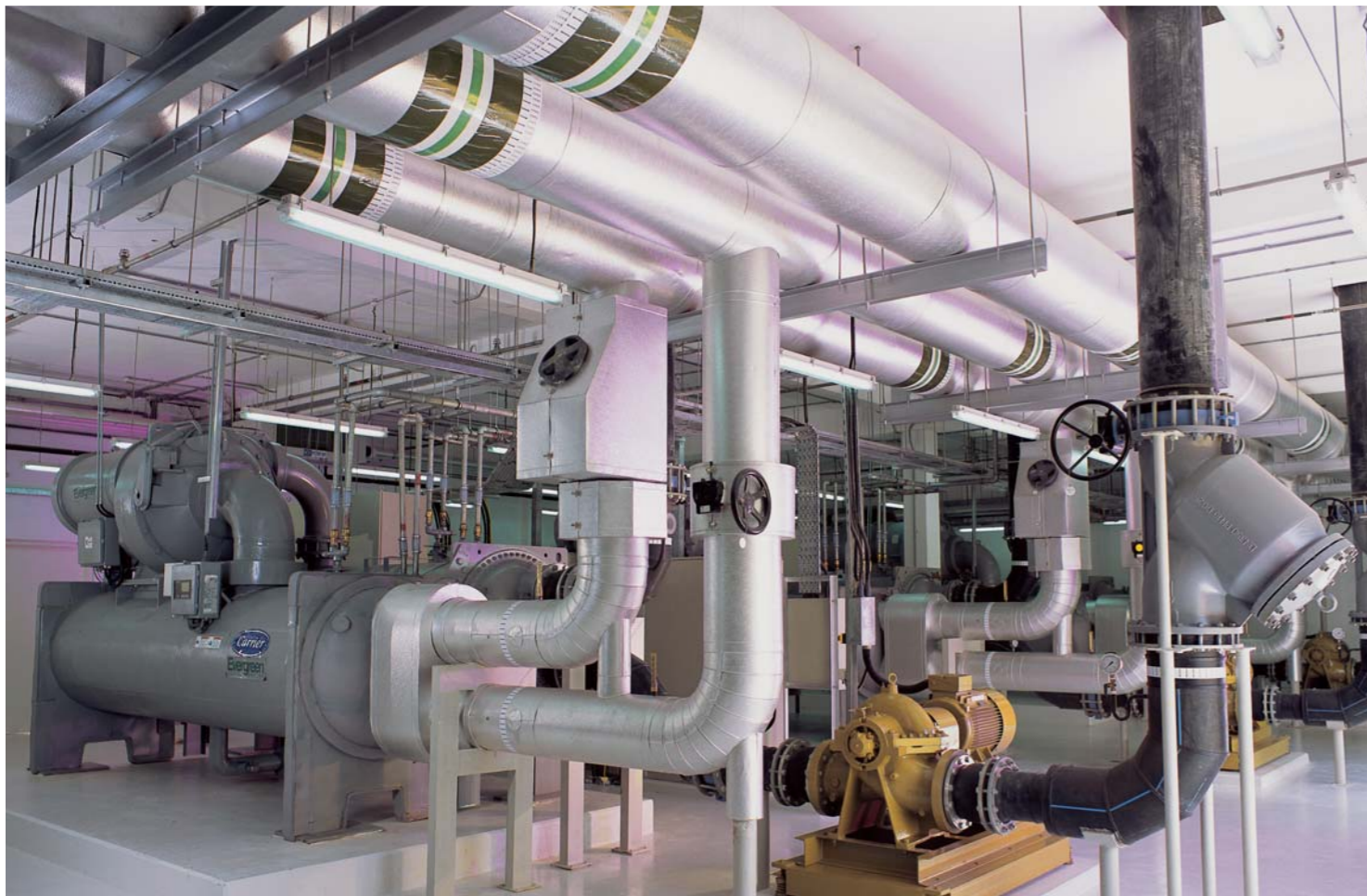
Water Cooled Centrifugal Chillers
