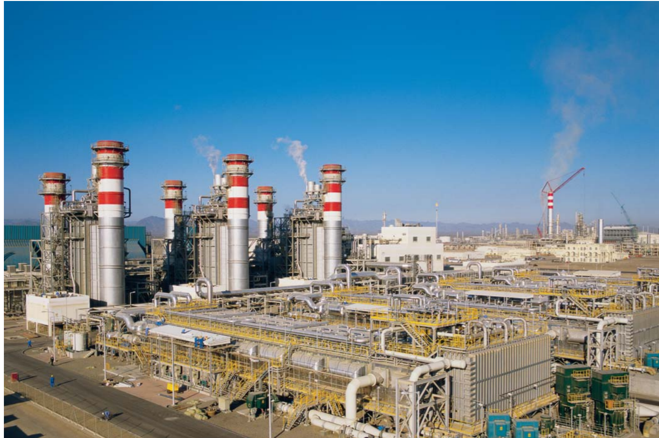
Mechanical, Electrical & Instrumentation construction for 585 MW Power & 33 MIGD Desalination, Sohar IWPP Phase-1 including 3 X 122MW GTG, 3 X 325T HRSG, 1 X 220MW STG and 33MIGD MSF Desalination Plant
