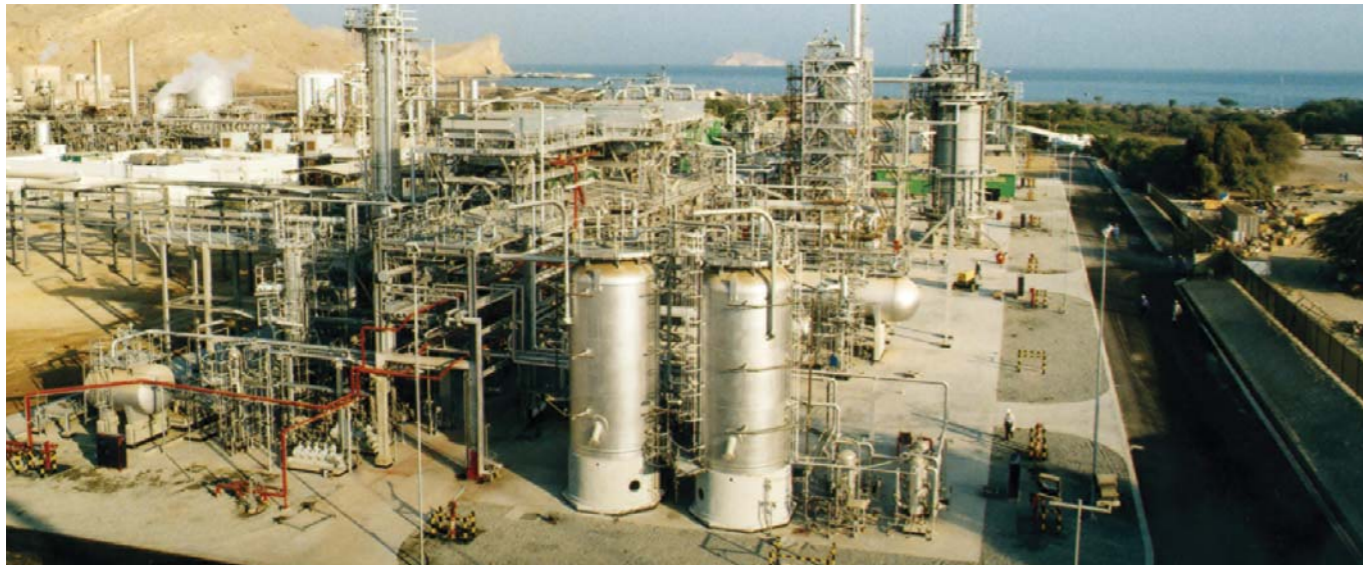
Complete Civil, Mechanical, Electrical & Instrumentation construction for DHDS Project, Oman Refinery
