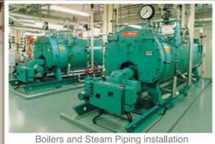
Boilers and Steam Piping installation
