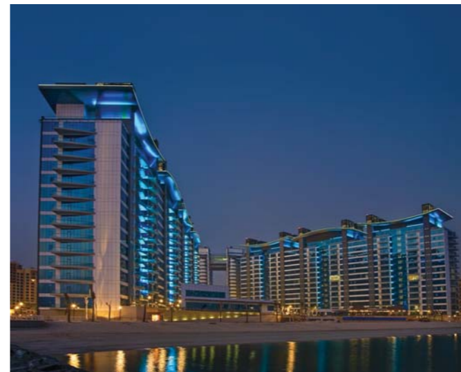
Movenpick Hotel & Furnished Apartments, Spa and 7 nos. Residential Towers for Oceana, The Palm - Dubai
