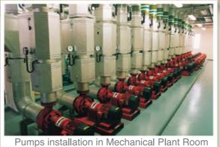
Pumps installation in Mechanical Plant Room
