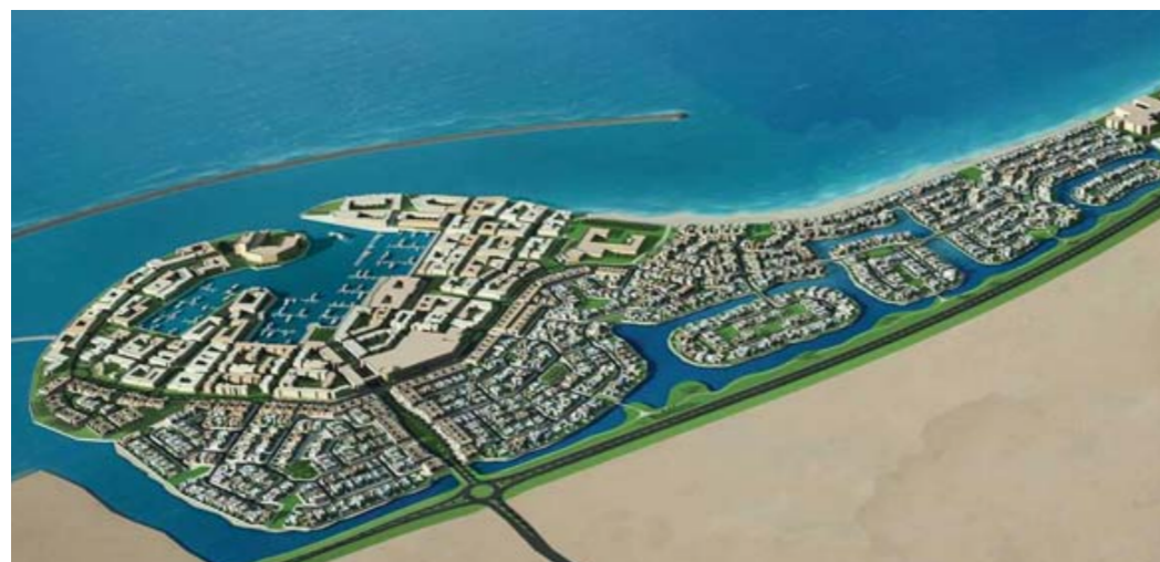
The Wave Muscat - District Cooling Plant.
