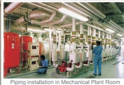
Piping installation in Mechanical Plant Room
