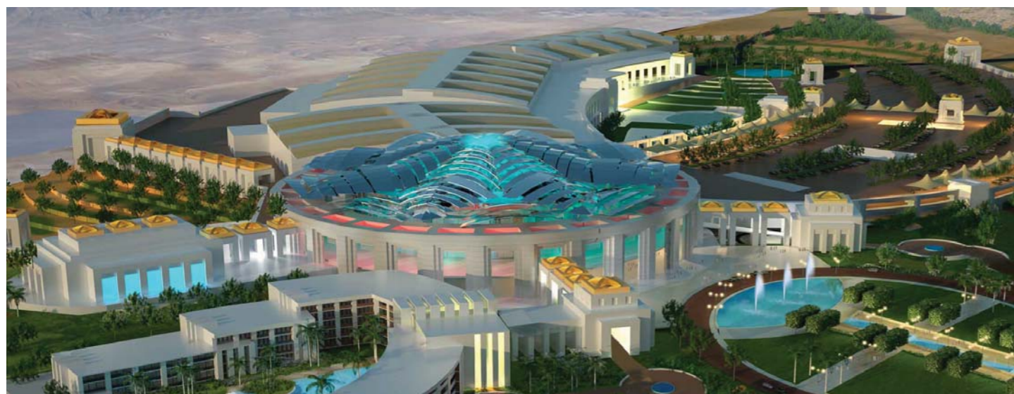
Oman Convention & Exhibition Centre, Muscat - MEP services for Exhibition Centre including centralized exhibition hall cooling Plant of 10000 TR.
