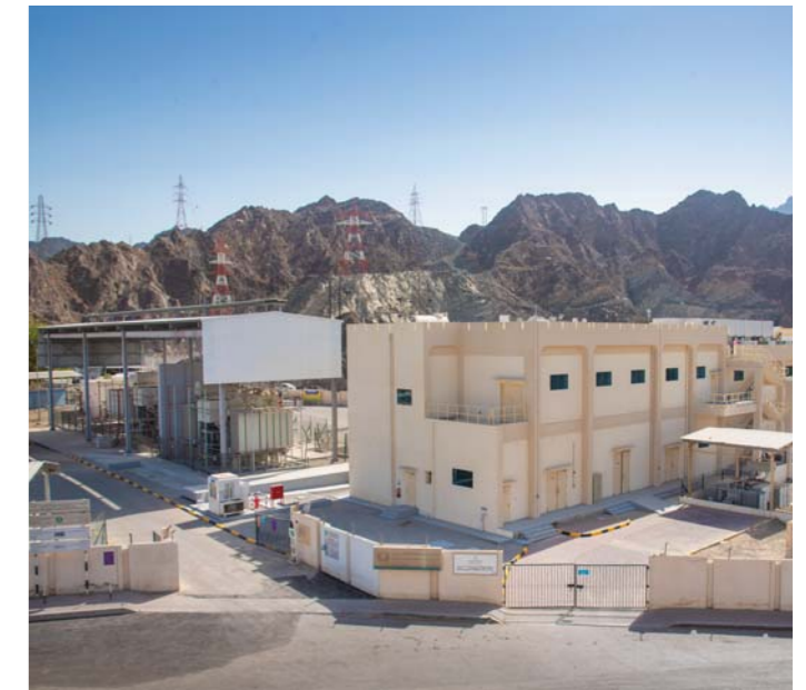
132/33kV Grid Station at Wadi Kabir
