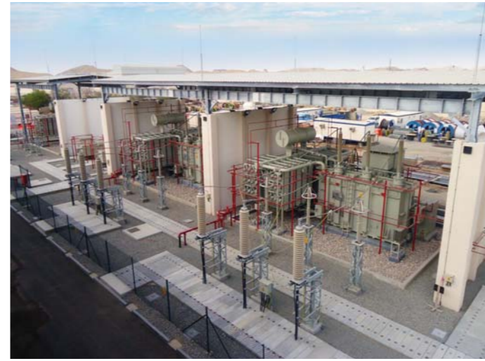
Construction of 132/33kV Grid Station at Rusail for OETC
