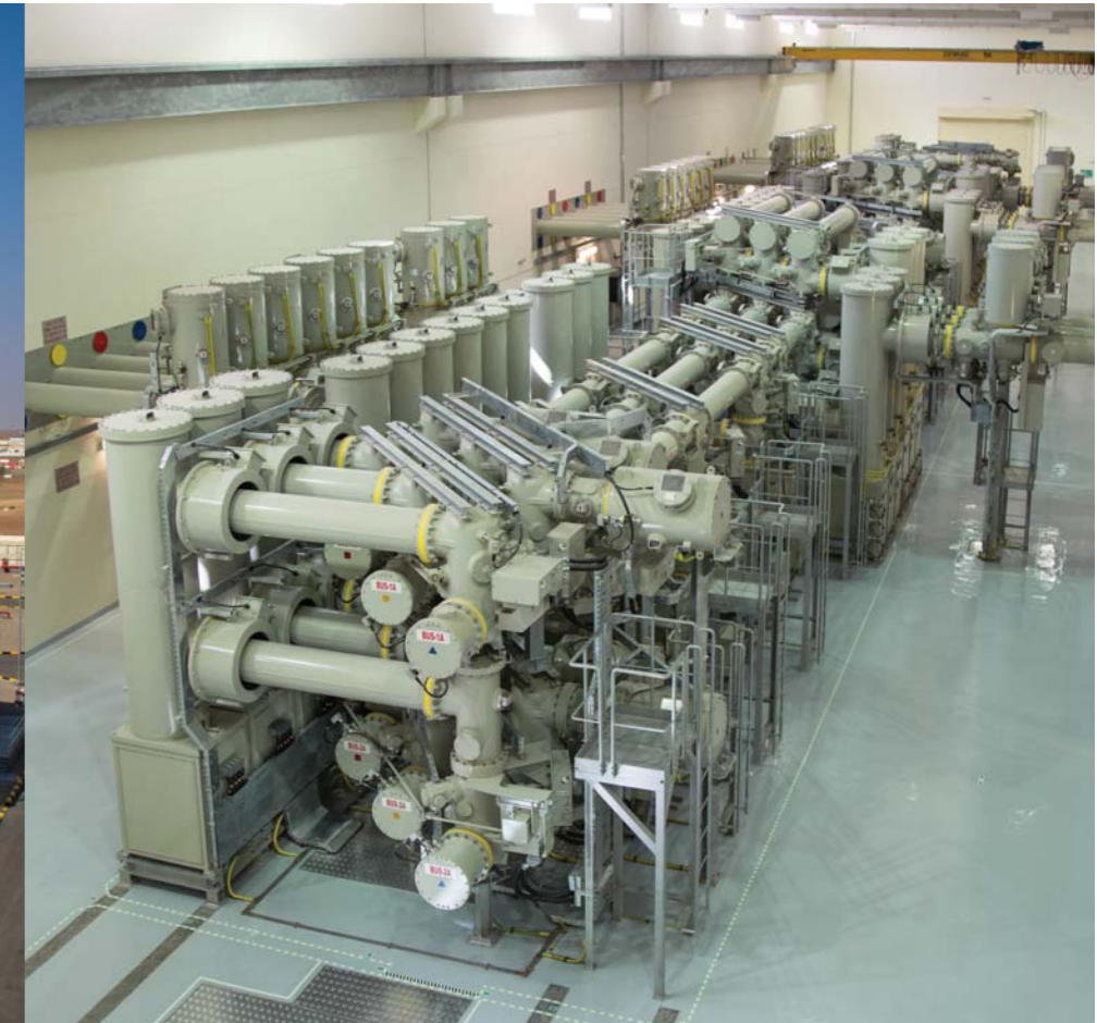
400kV GIS – 17 Bays with Bus Duct, 3x500MVA Transformers for New 400/220kV IPP Grid station at Ibri, Oman
