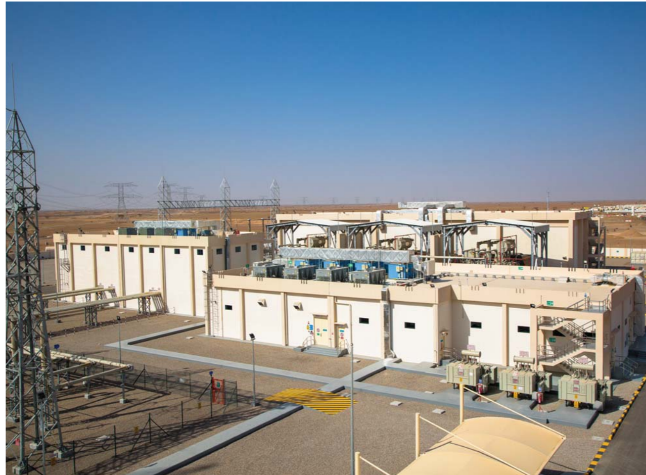
400kV GIS – 17 Bays with Bus Duct, 3x500MVA Transformers for New 400/220kV IPP Grid station at Ibri, Oman
