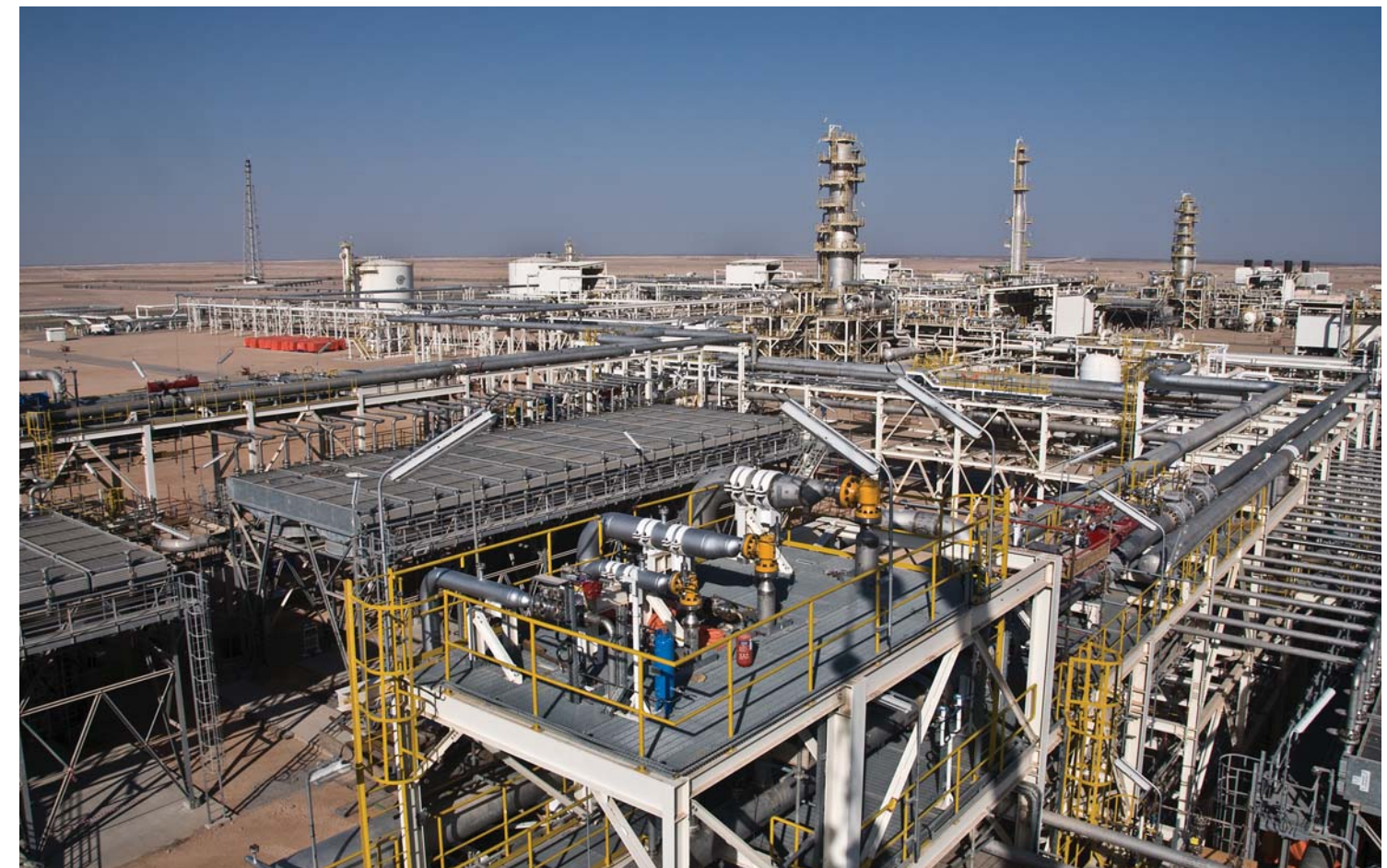
A view from the Pipe Rack
