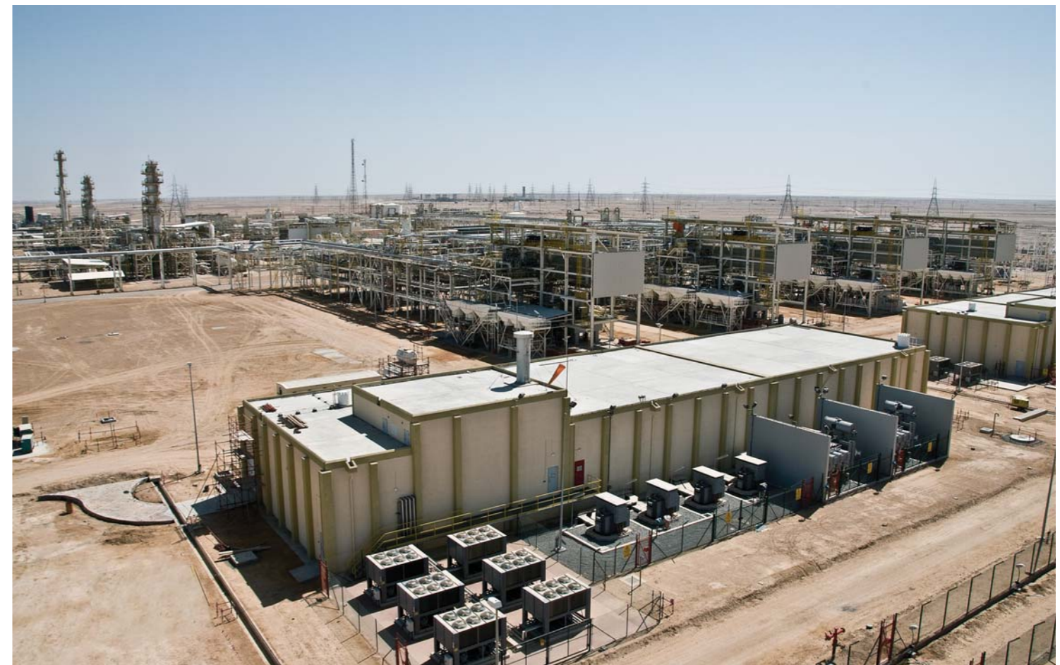
Aerial view of Compression Plant
