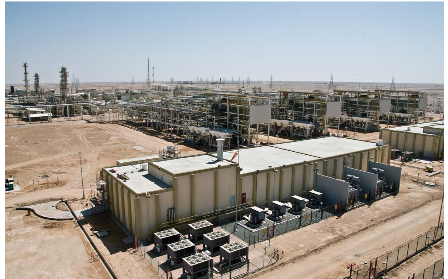
Aerial view of Compression Plant
