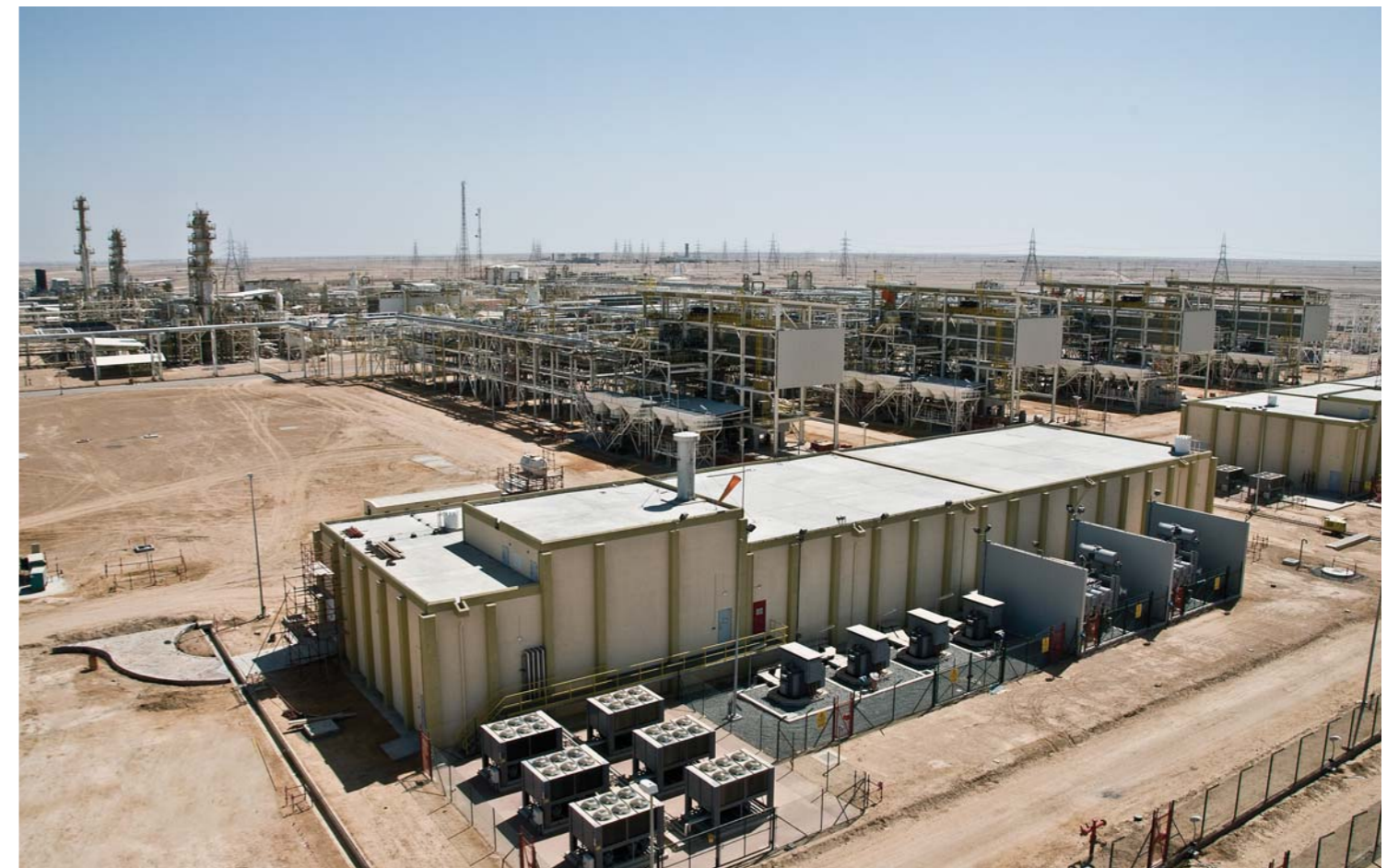
Aerial view of Compression Plant
